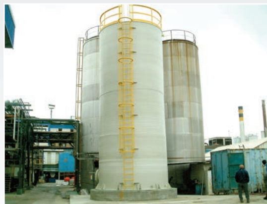
10,000 gallon PP tank featuring seismic design, OSHA compliant ladder, safety cage and handrails.
