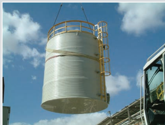
Crews prepare to install a 13.2’ diameter, 15,000 gallon flat bottom PP tank equipped with OSHA compliant ladder, safety cage, and handrails.
