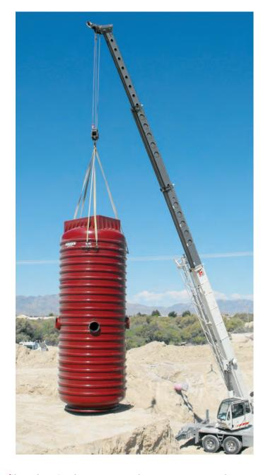
tural strength. Because the integral ribs and tank are made of the same materials — high-quality resin and glass — and are manufactured as a monolithic structure, Xerxes products, whether installed vertically or horizontally, are very robust vessels.
