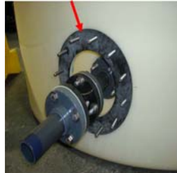
Install Outer Face Plate and SS Back Ring
