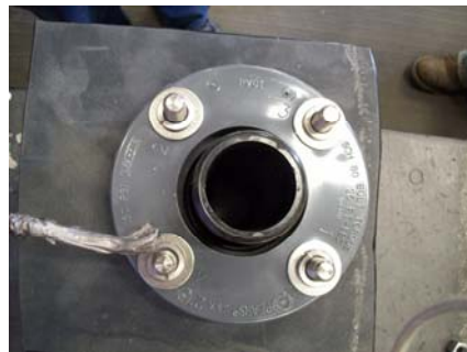
Add flat and lock washers, apply a small amount of anti-seize compound, and screw the nuts onto the studs
