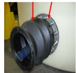
Install bellows and SS Back Rings
