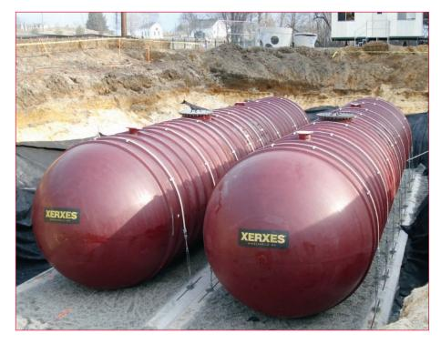
have sewer and water was challenging in a site with "little room to manipulate the parts," Murphy continues. The CVS project required a 50,000-gallon-capacity system for nonpotable fire-protection water.
